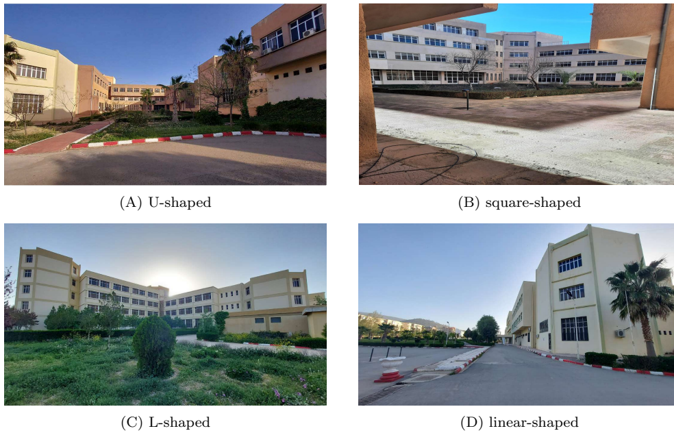
FIG. 2. Photographs of each measurement stations.
