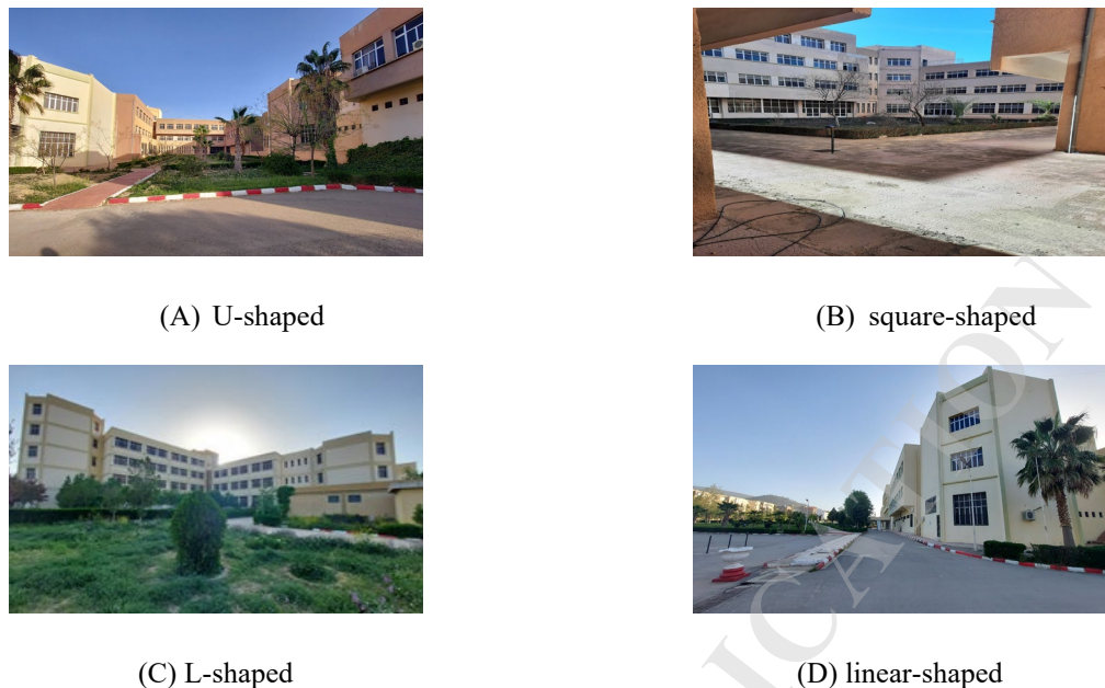
Fig. 2 Photographs of each measurement stations.
