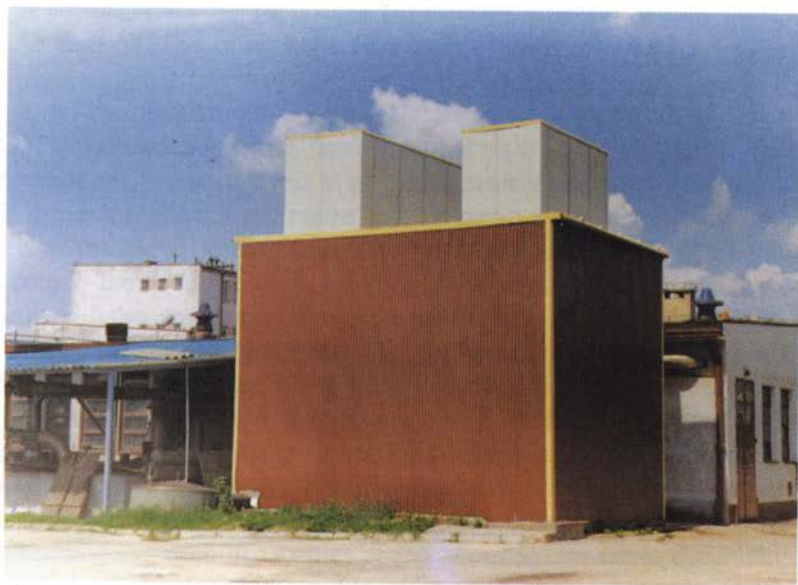
Fig. 4. Entirely closed enclosure (with noise dumpers on the exhaust holes) protecting the unit of two condensers in the Okręgowa Spółdzielnia Mleczarska in Pajęczno.
